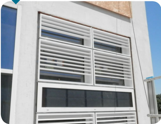
Multifunctional façade energy prototype installed on the laboratory building of ACCIONA in Sevilla (Spain)
